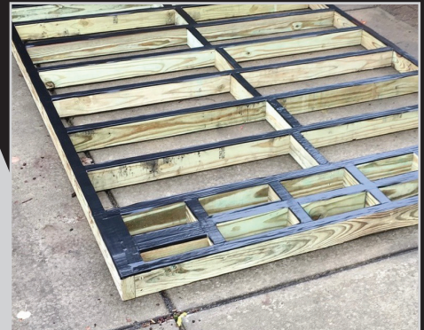
Photo: Courtesy of @alfanoconstruction
