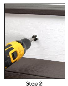
Drill 1" diameter hole through riser for recessed light using 1" forstner drill bit.
