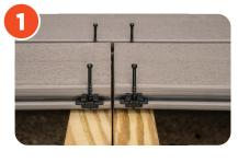
Place 4 clips centered on joist on both sides of the boards.
