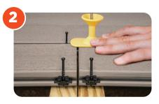
Place the next board up against the clips then fasten the screws.
