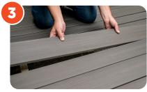
Clean away any clips remaining on the joists and lay the new deck board in position without any clips in place.
