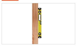
Make final adjustments to pergola positioning, using a level to plumb posts.
