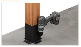
Predrill holes for anchors using a %6" concrete drill bit. Install provided screw anchors to secure pergola to concrete.
