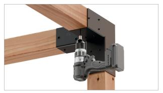
Install all screws into connector on each end of beam. Repeat Steps 5 and 6 for remainder of beams. Remove temporary bracing.
