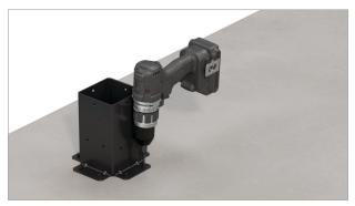
Predrill holes for provided anchors using a %6" concrete drill bit. Install provided screw anchors to secure pergola to concrete.
